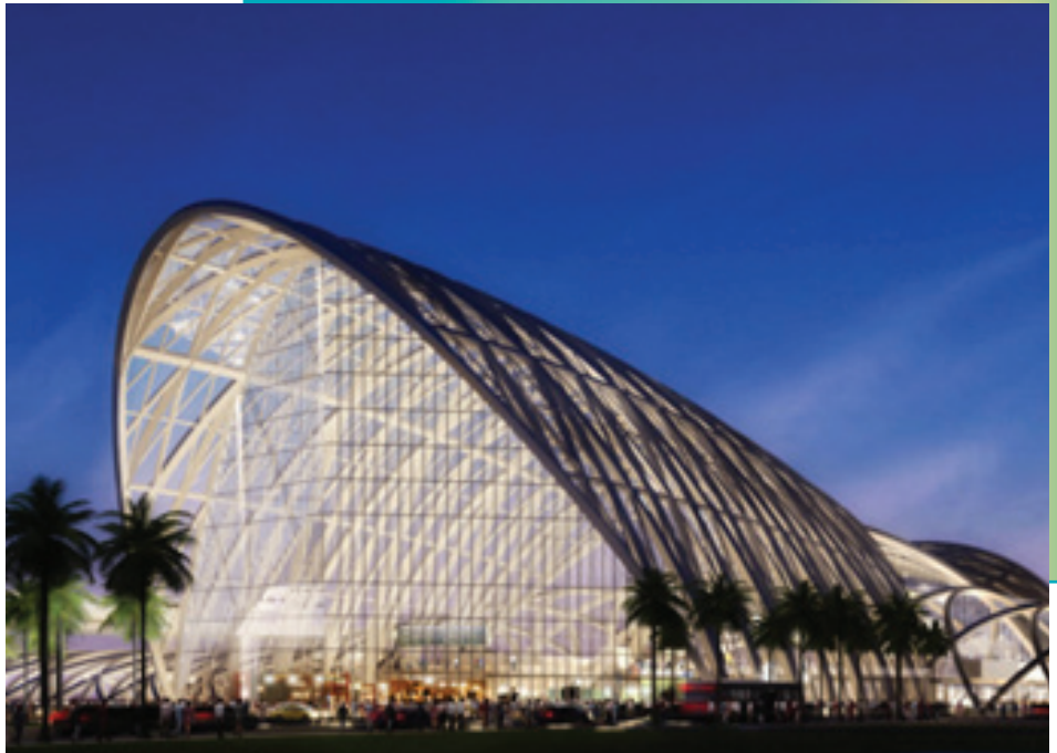
Anaheim Regional Transportation Intermodal Center – ARTIC
