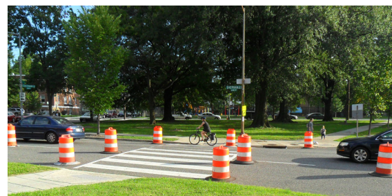
VHB designed bike lanes for Sherman Circle NW in the District of Columbia, which were tested using temporary traffic control devices as part of a tactical urbanism pilot and then permanently implemented by DDOT.
