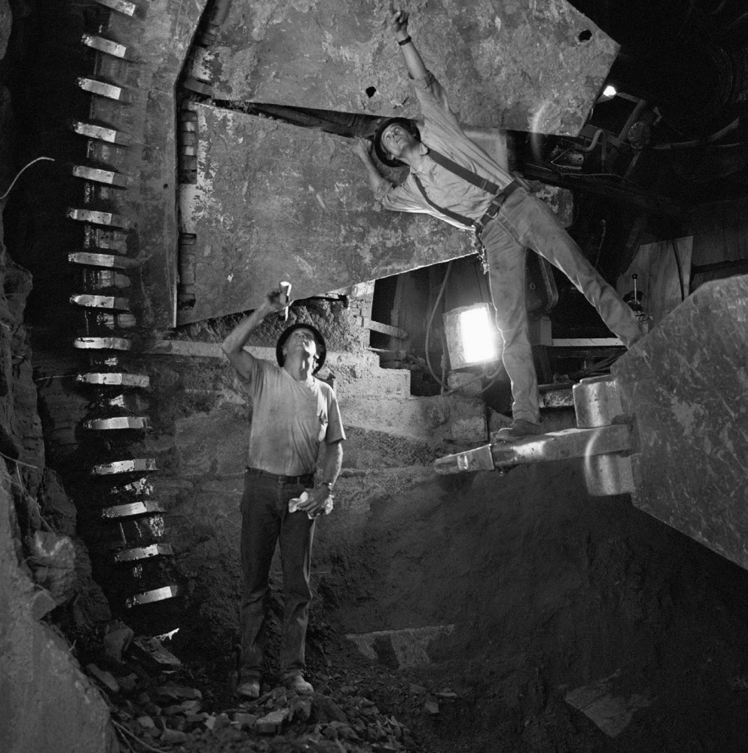
Two miners inspect the breasting plates and teeth of the shield machine soon after it broke through to the station at 6th St and Vermont St. Two tunnels were bored underground from the construction site at Barnsdall on Hollywood Bl.
