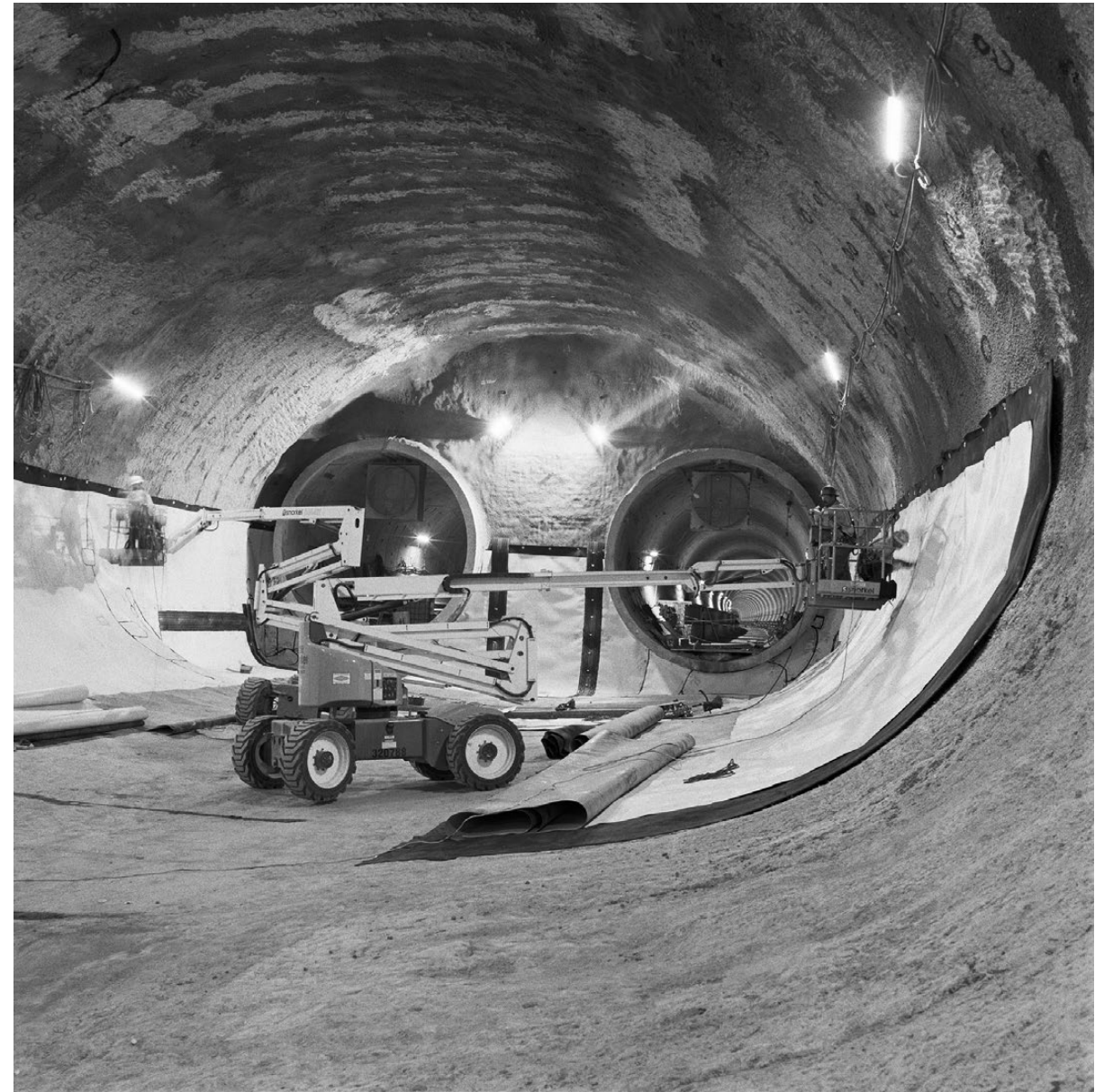
Workers install waterproof lining on the shotcrete lining surface of the Rail Crossover Cavern prior to the final lining installation.
