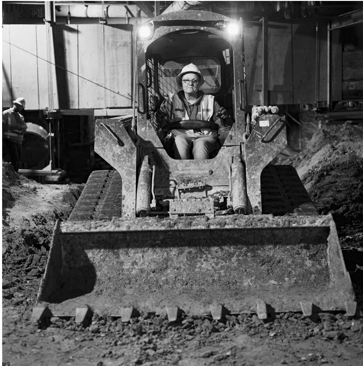
Lori Douglas, Heavy Equipment Operator, is removing the dirt for the “cut and cover” section of tunneling on the Regional Connector project.
