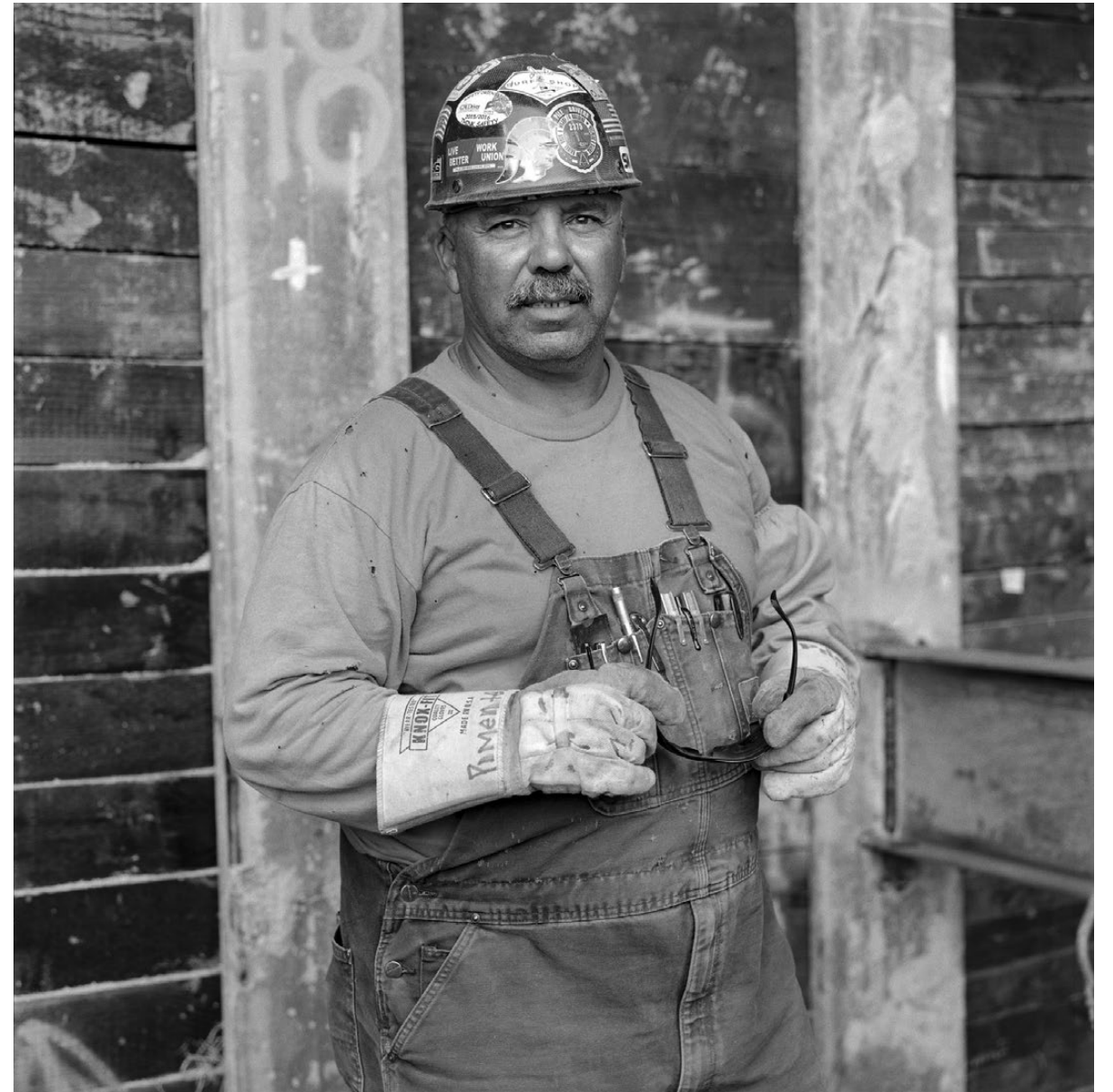
Ralph Pimentel, Carpenter, poses at the future station. Pimentel was welding the tieback anchors 110' below street level, making it the deepest point in the Metro system.
