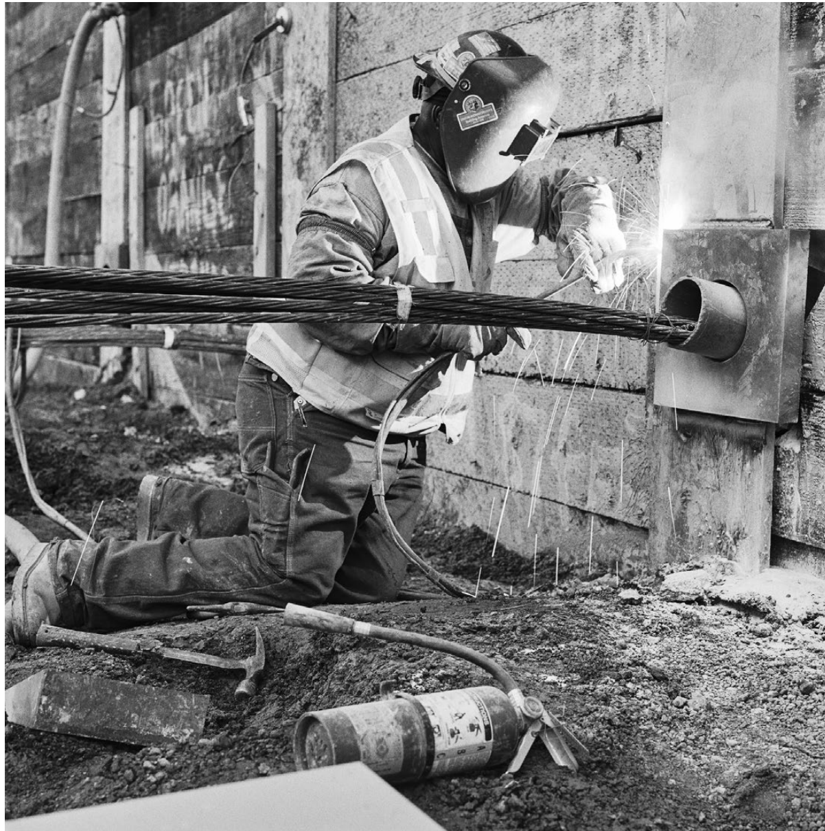
Karagozian relays, "A construction worker welding can make for a dramatic long exposure photograph. Here the worker is welding a tieback anchor collar to a soldier pile."
