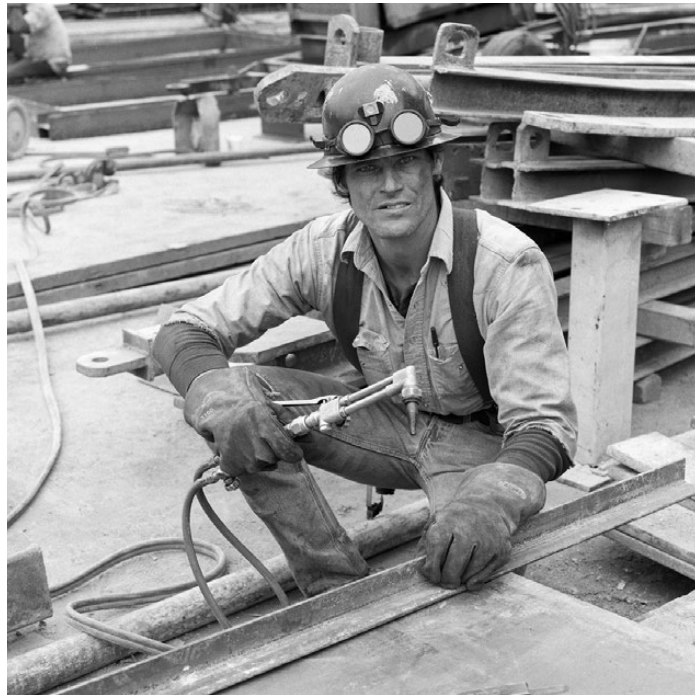
Pictured here at the Barnsdall topside construction site, Tony Anderson, a Tunnel Equipment Operator, worked many different tasks for the Red Line project from mining to welding, and as a mechanic.
